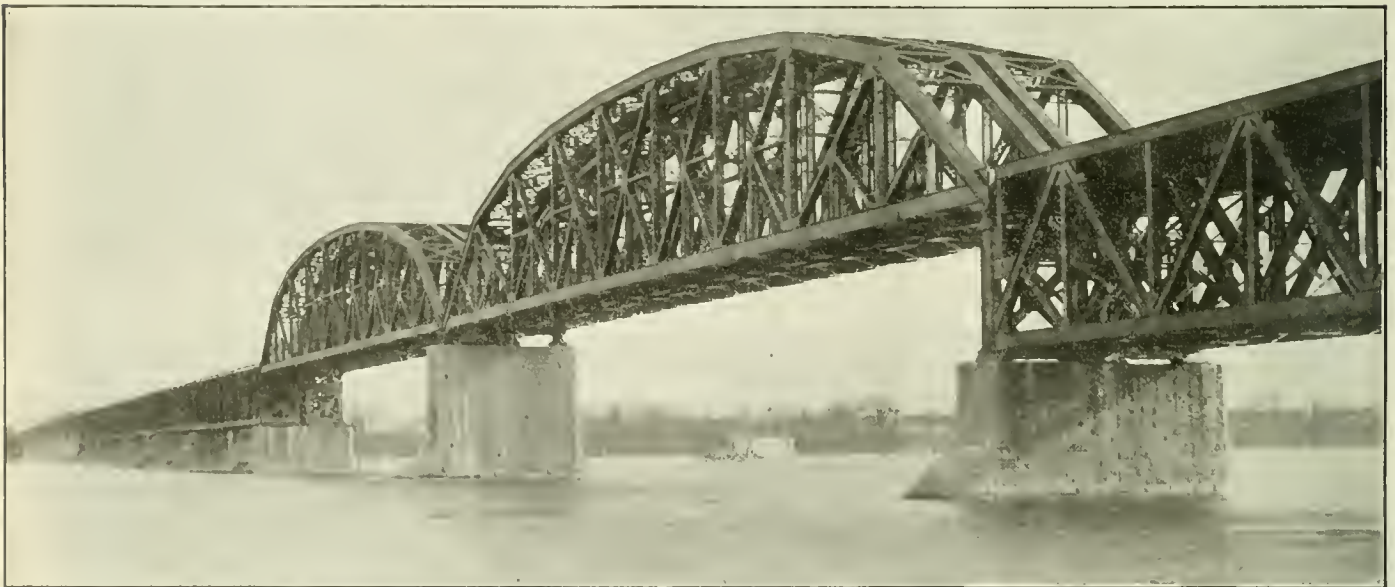
THE CHANNELED SPANS OF THE ST. LAWRENCE RIVER BRIDGE.
